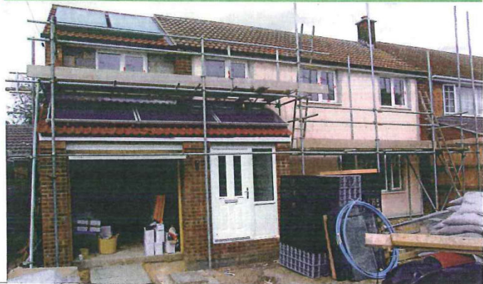
One of two properties acquired by Huntingdonshire District Council as part of BRE's Rethinking Refurbishment project
